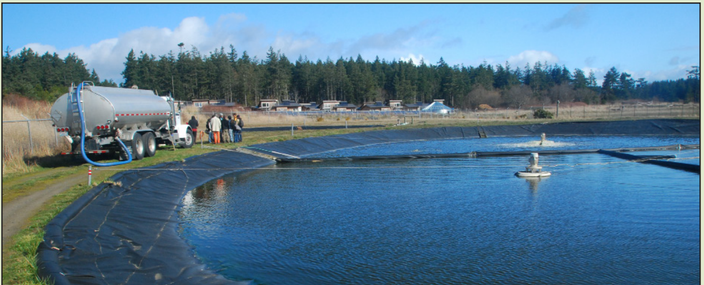
Fisherman Bay sewage treatment facility.
