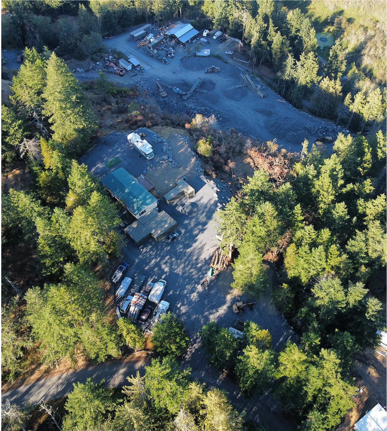
This is an overview of the Egg lake Quarry and the residential parcel noted here.
